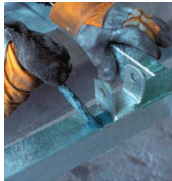
Approved epoxy-based zinc-rich paint is applied to the uncoated area to at least equivalent thickness to the galvanized coating.
