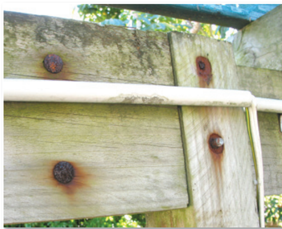
CCA treated pine is very aggressive on both zinc and steel when its moisture content exceeds 20%. These electroplated bolts have almost totally corroded in pergola structure after 10 years.
