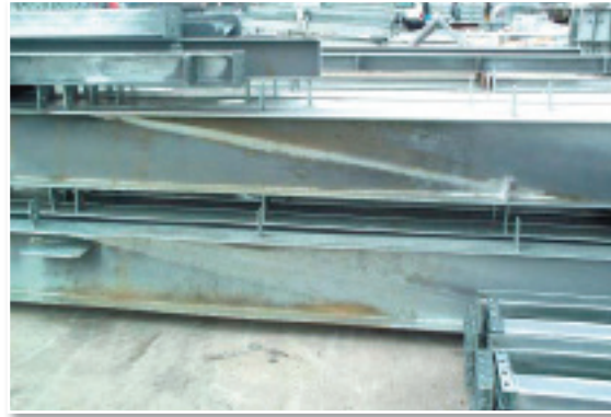
This long universal beam has been double dipped, leaving an aesthetically unacceptable double-dip mark on the beam. This can be avoided by sizing sections to single-dip dimensions.
