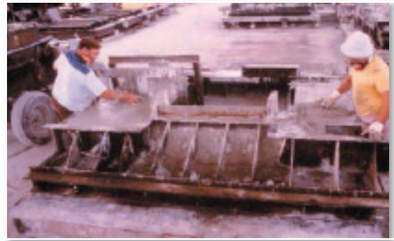
Galvanized reinforcing bar is widely used in the pre-cast concrete industry because the elements are almost always used as exposed facades and concrete cover is limited by design.
