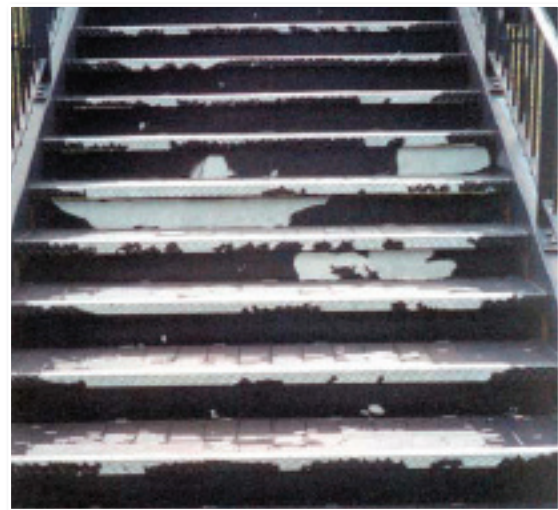
Complete failure of this paint system on this galvanized stairway occurred because the paint was applied directly to the chromate quenched galvanized surface. This passivation treatment interferes with paint adhesion
