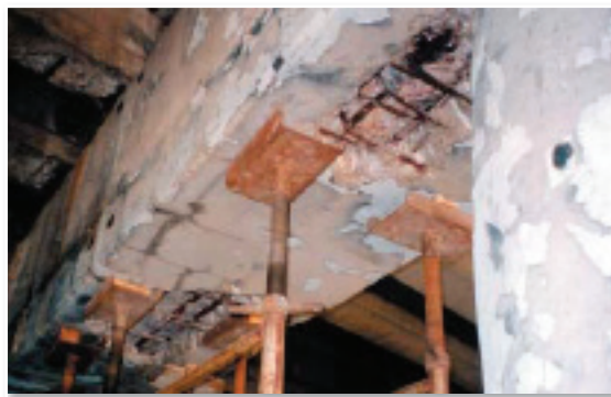
The corrosion of the reinforcing bar in this road bridge in North America has occurred because of poor rebar placement combined with the use of de-icing salts on the road.
