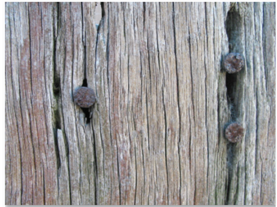
Uncoated steel nails used in hardwood not only corrode themselves by the corrosion products attach the surrounding timber
