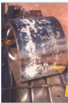
White rust on newly galvanized guard rail section caused by nesting items in wet conditions.
