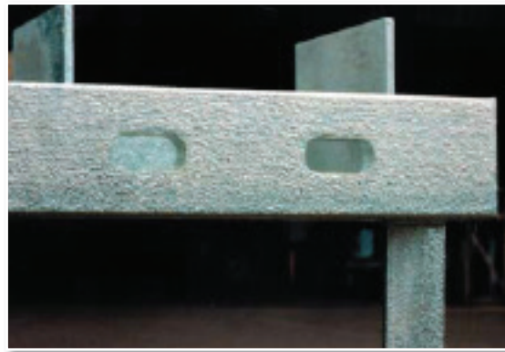
The textured surface on this steel angle results from the rough as-rolled surface of the base steel, usually caused by excessive mill-scale on the steel section in the hot rolling process.
