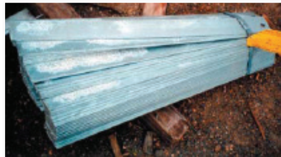
The 'white rust' on these galvanized flat bar sections has been caused by their being wet in the bundle. Galvanized coatings require good ventilation when newly applied to allow the passive oxide films to develop.
