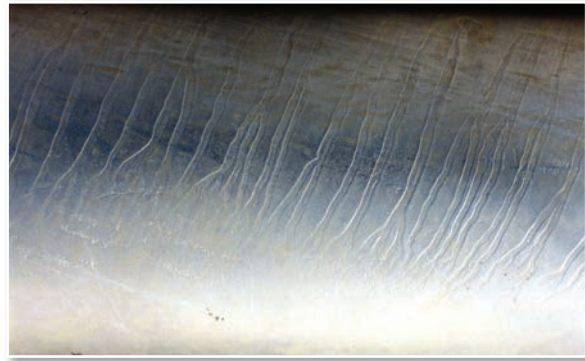
Fishbone striations on large diameter pipes arise from surface stresses in the steel causing different zinc-steel reaction rates on the pipe surface.
