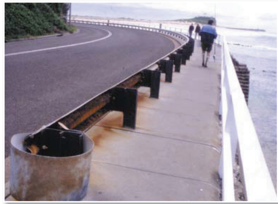
Severe marine environments such as this ocean front site may have zinc corrosion rates of around 20 microns or more per year. In this environment, the galvanized coating on the guardrail has a predicted life of 3-5 years.
