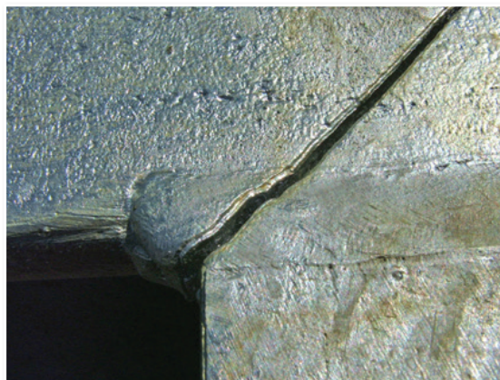
Crack propagated from the corner of this angle frame after galvanizing is suspected of arising from liquid metal assisted cracking.
