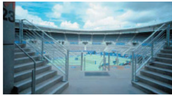
The Sydney Olympic Tennis Centre was specified INGAL SSQ – Special Surface Quality – for this important sporting facility.
