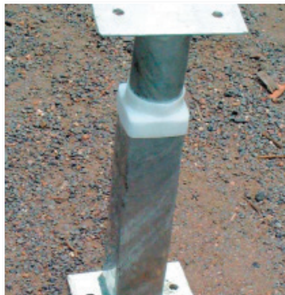
Continuous galvanizing processes have been developed for a large range of smaller hollow sections. Some are galvanized externally only and typical coating thickness is approximately 20 microns.
