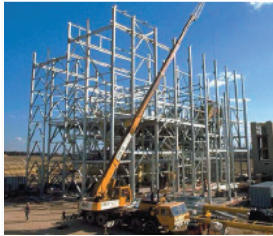
Industrial facilities like this coal treatment plant at Teralba, NSW process 800 tph of coal 24 hours/day, 7 days/week. The cost of down-time for coating maintenance is a bigger factor than coating cost.
