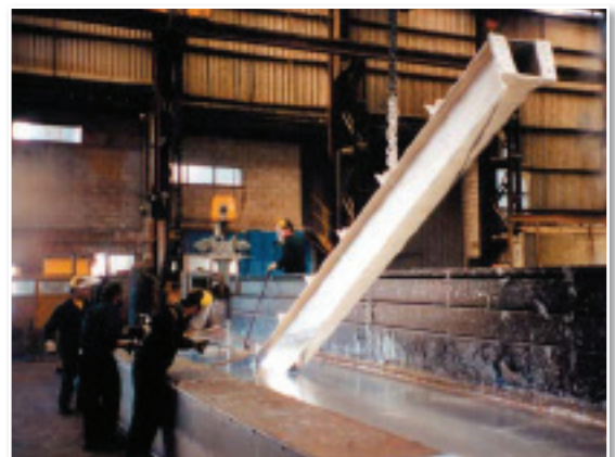
By lifting long items in chains connected to cleats or lifting lugs allows steep withdrawal angles and avoids chain touch marks on the fabrication.
