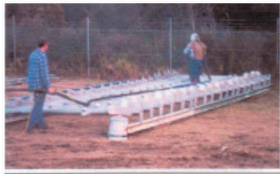
These galvanized conveyor frames are being brush-blasted prior to the application of a heavy-duty paint coating. This is a very effective surface treatment for painting over galvanized surfaces.
