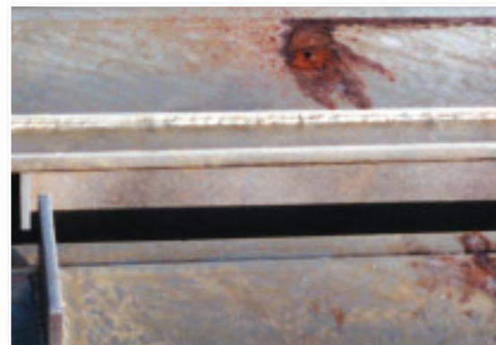
Flux staining has occurred on unsealed vent holes in overlaps on this fabrication. The stains are caused by iron salts, that have penetrated the overlap during pre-treatment, re-hydrating with atmospheric moisture.
