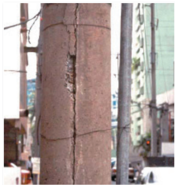
The corrosion of the steel reinforcement in this concrete power pole has cause it to split from end to end.
