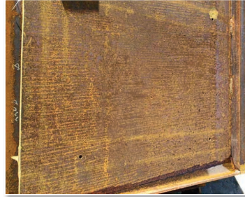
Steel must have an anti-corrosion coating for most external applications and ensuring long service life for steel enhances its environmental credentials.
