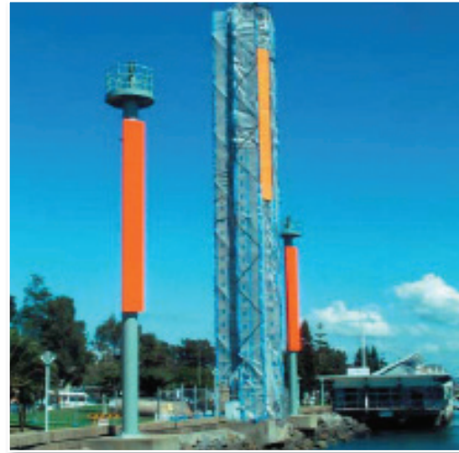
Environmental controls are much more stringent where maintenance painting is required, even for non-hazardous coating. This navigation tower required full containment for its refurbishment.
