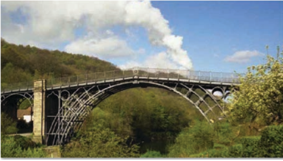
Iron Bridge, completed in 1779, was built using concepts found in carpentry – including mortice & tenon and blind dovetail joints.
