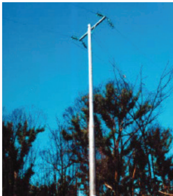
Galvanized coatings slowly weather away, with the zinc ending up in the soil. Most soils are zinc deficient and this has no negative environmental impact in most instances. All protective coatings prolong the life of steel and make an energy saving contribution as a result.
