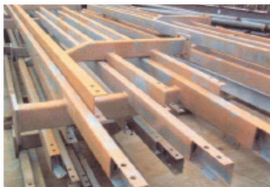
These steel bridge railings have been abrasive blasted prior to coating but have flash-rusted, requiring further surface treatment prior to coating
