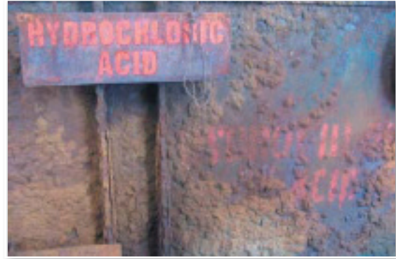
Difficult surfaces such as the corroded steel shell of the hydrochloric acid pickling tank require stringent surface preparation to remove both corrosion products and residual chlorides
