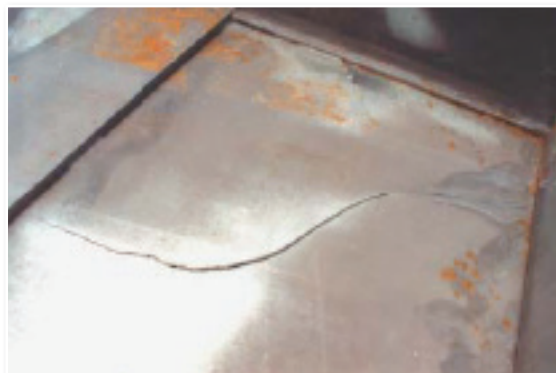
This fracture in high-strength Bisalloy plate resulted from hydrogen embrittlement induced by the acid pickling process. High strength steels such as this can be satisfactorily galvanized by mechanically cleaning the surface and avoiding the acid pickling pre-treatment stage in the galvanizing process.
