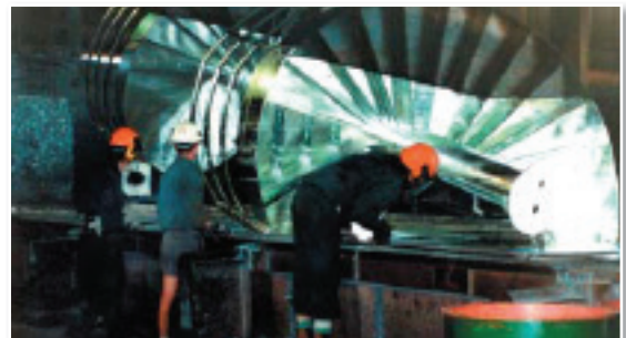
Large and complex fabrications can be hot dip galvanized by double dipping. This large spiral staircase is half-way through the dipping process.
