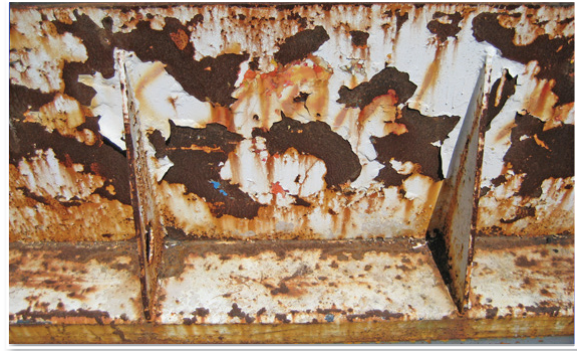
Poor quality paint systems can accelerate steel corrosion by concentrating pollutants and corrosion cells around and under the paint film.
