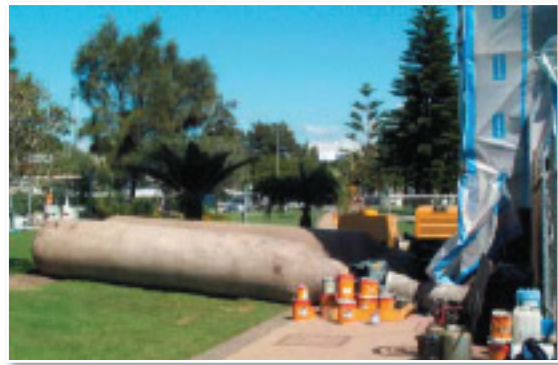
EPA requirements on some repainting projects require full filtration of the extracted air.
