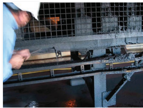
These galvanized conveyor stringers have been largely unaffected after being covered in coal spillage for over 10years at North Goonyella.
