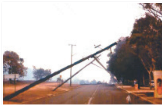
Timber poles following grass fire in ACT in 2003 – burnt off at base
