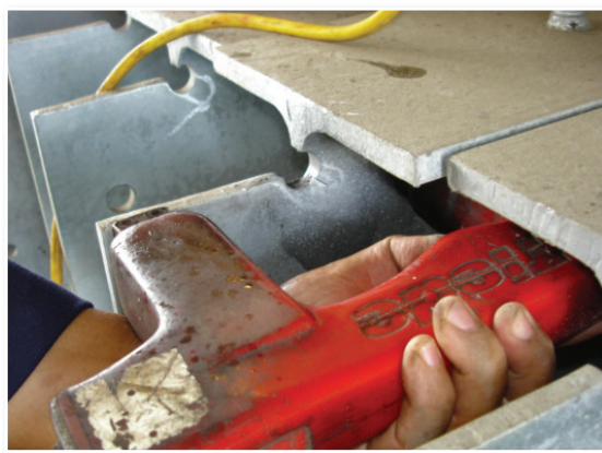
These large galvanized beams, galvanized in Malaysia, have all been affected by 'cope cracking' in the circular (coped) area of the beam webs. Steel sourced from electric furnace sources is more prone to this form of liquid metal assisted cracking than steel sourced from blast furnaces. This phenomenon has never been reported in Australia as all the locally produced structural sections are manufactured from blast furnace sources.
