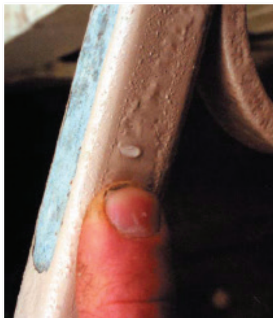
Poor surface preparation (no primer used) combined with paint application on damp galvanized steel resulted in this paint failure caused by water blisters under the paint film.
