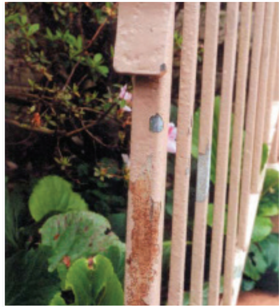
Paint failure on galvanized balustrade resulted from paint being applied to a contaminated surface.
