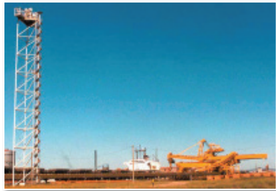
This navigation tower on Newcastle (NSW) Harbour was galvanized and painted to provide additional durability in a marine environment, and remains in good condition after 20 years in service
