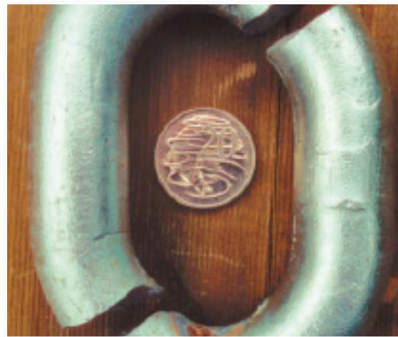
Hydrogen embrittlement failure of Herculloy chain is caused by exposing this 1200 MPa steel to pickling acid. These types of steels should not be galvanized.
