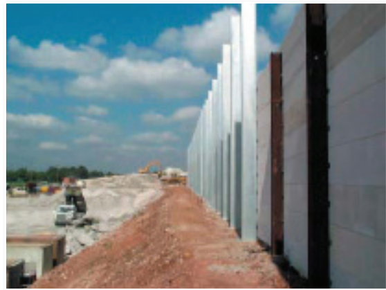
The galvanized steelwork supplied by Industrial Galvanizers to the M5 East Motorway project for the NSW Roads and Traffic Authority in 2003 has a 25 year coating guarantee
