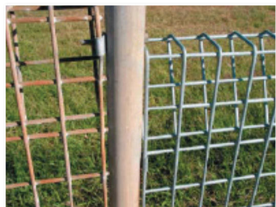
These old (l) and new (r) fence panels show the life cycle of a galvanized coating. Galvanized coatings are slowly eroded by oxidation of the surface. The oxidised lower layers of the zinc-iron alloy layer of the galvanized coating indicate that the coating is nearing the end of its life.
