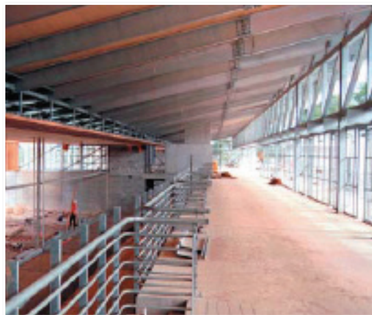
The Sydney Olympic Shooting Centre is an excellent example of a significant bolted galvanized structure where fast erection and low long-term maintenance were a requirement of the design.
