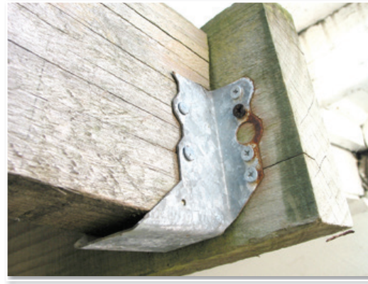
Poor performance of the single electroplated fastener in this external hanger bracket, compared to the galvanized nails after 5 years in treated pine.
