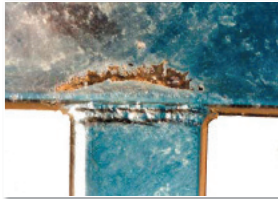
This miss in the galvanized coating is caused by surface contamination by residual oxides not removed in the pickling process.
