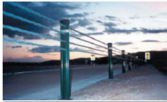
INGAL Civil Products is a division of Industrial Galvanizers that powder coats all its galvanized Flexence roadside safety posts with 100% reliability
