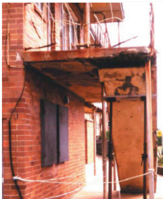
Corrosing reinforcing bar has caused severe spalling of the concrete on this oceanfront dwelling.
