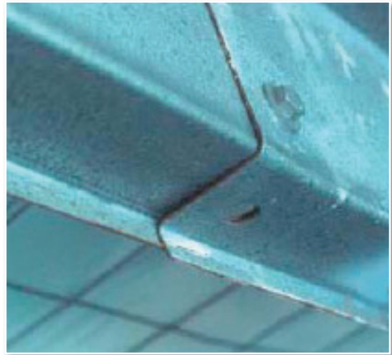
Pre-galvanized products rely on cathodic protection to prevent corrosion on their cut edges. Thicker sections such as these heavy purlins are on the borderline and corrosion is visible on installation.
