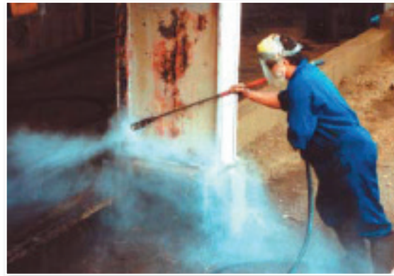
Ultra-high pressure (35,000 psi+) water blasting is an effective way of preparing contaminated surfaces for maintenance painting, particularly where chlorides are present.
