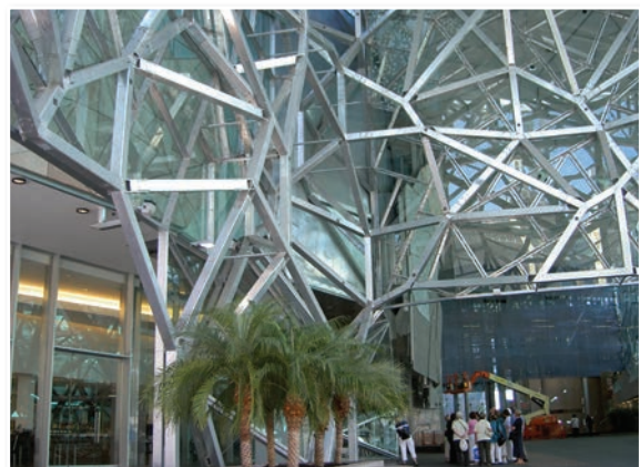
Federation Square, Melbourne: galvanised interior AESS. Given the height of the building, most of the sections and joints are more than 6m away from the viewer. A different AESS standard can be applied compared to steelwork at ground level, which is highly visible.
