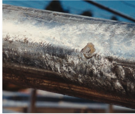
Where jigs are used to support large items in the galvanizing processes, touch marks will occur where the galvanized coating adheres to the jig at the point of contact.
